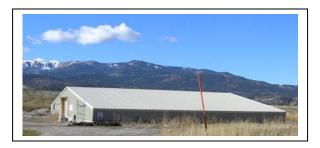
The wastewater treatment system includes "....two packaged treatment plants, one rated at 25,000 gpd and one rated at 65,000 gpd. Currently only the 65,000 gpd plant is in operation. The 25,000 gpd plant is useable with some improvements for treatment of raw wastewater or as an aerobic digester for the waste biosolids from the 65,000 gpd plant" (Nelson Engineering, 2006).
